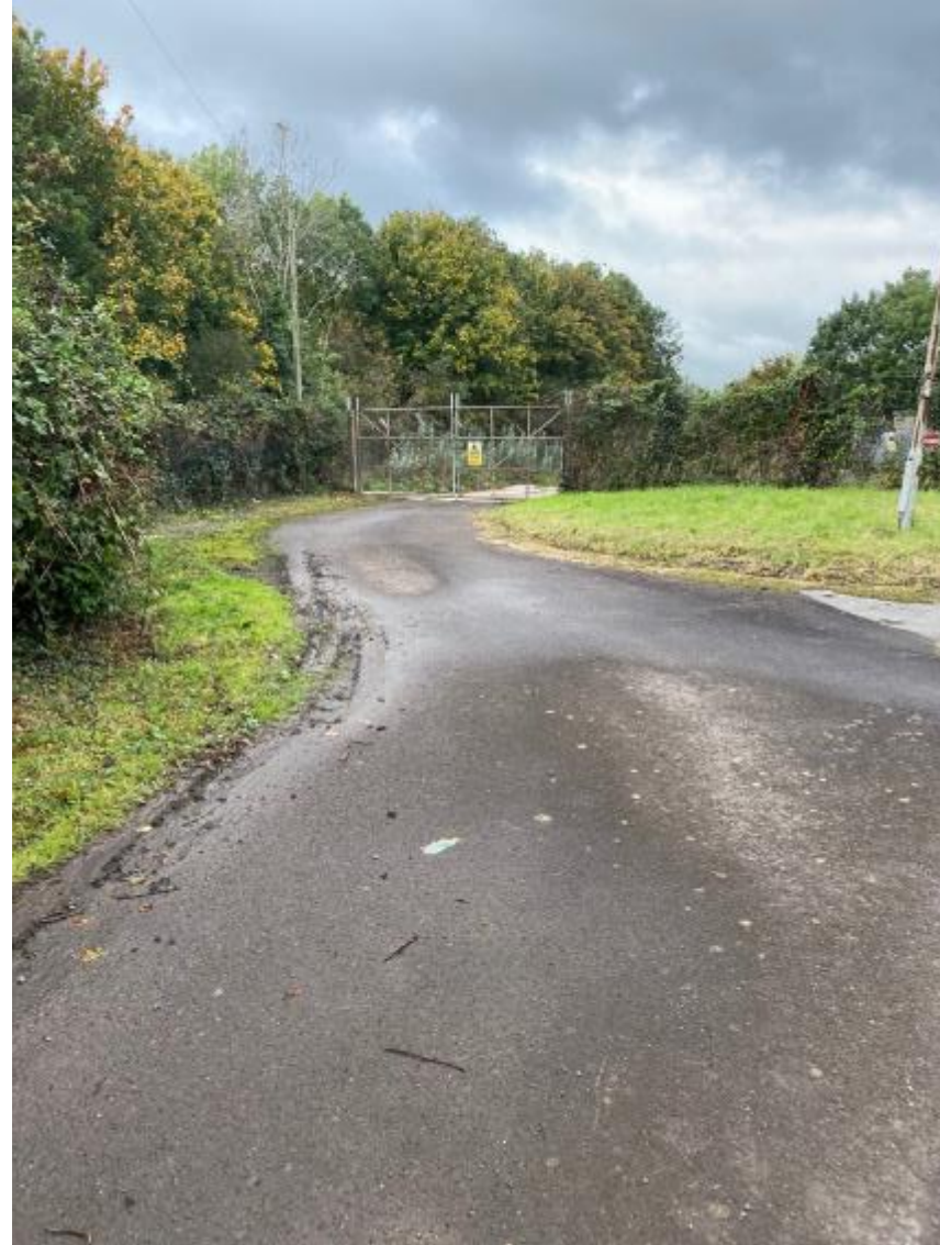
Gates at entrance to site
